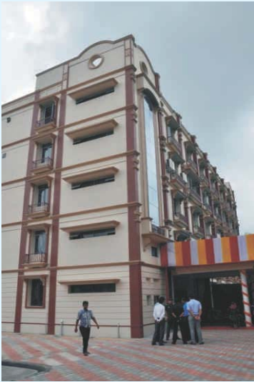
New Building of Area Accounts Office, Kolkata, LAO (A) (B) (C) (D) & RAO (MES), Kolkata
